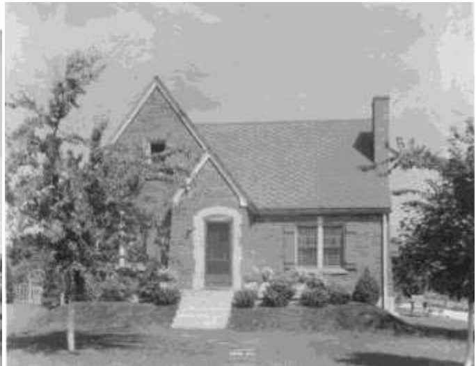
3705 St. Germaine Ct. constructed in mid 1930's and sold for around $9,000.00 sold in 2006 for $345,000
