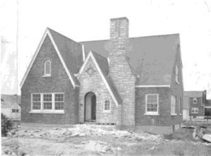
House under construction at 3815 St. Germaine Court
