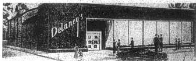
Papers were signed Friday through which the DeLaney Furniture Co. leased the above pictured building now under construction in St. Matthews, from the Wakefield - McMakin Realty Co., owner of the property. C. W. Jennings, of the Dahlem Construction Co., will supervise the construction.
